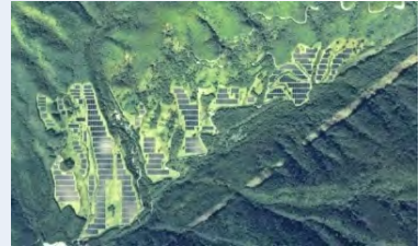
Environmentally sustainable photovoltaic power plant (image) Forum for East Japan Smart City Project / Meidensha Corporation
