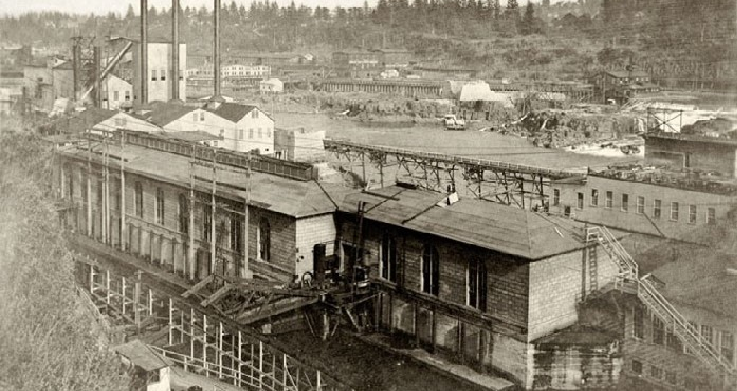
Electric power generated by hydropower
