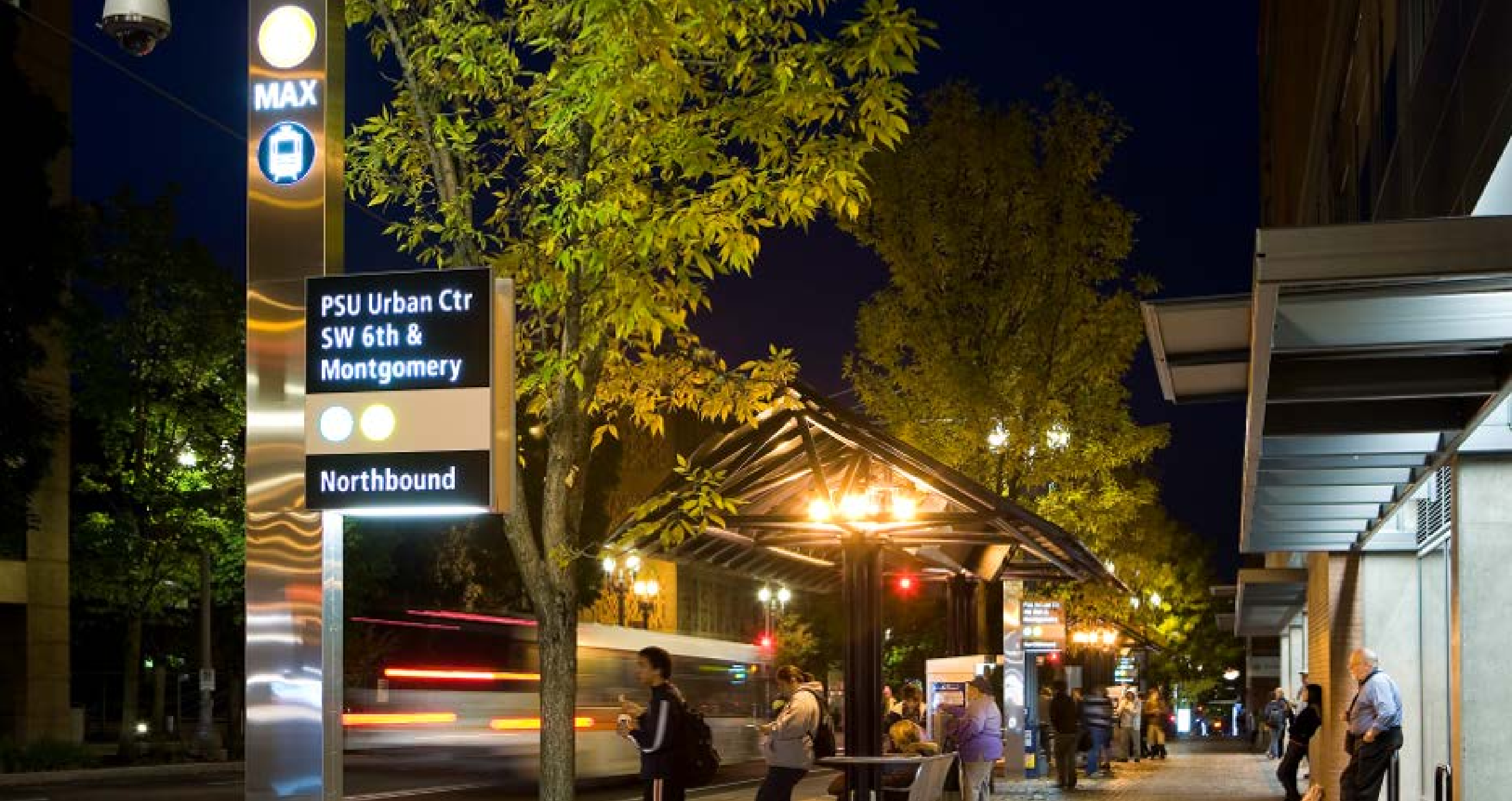
2009: Green Line Light Rail – Portland Mall Revitalization project
