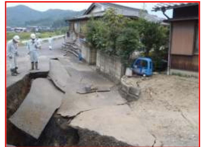
(Photograph: Damage caused by massive ground subsidence which occurred in October 2010)
