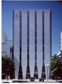
The Taisei Sapporo Building, which achieved a 52% reduction in CO 2 emissions
