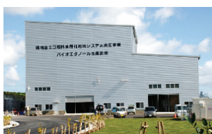
<Bioethanol production facility>
