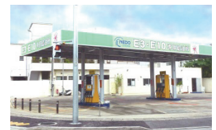
<Bioethanol supply facility>
