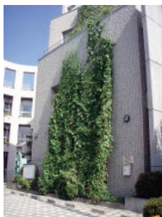
〈Installation of green curtains at public facilities〉
