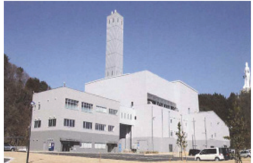
Waste disposal center
