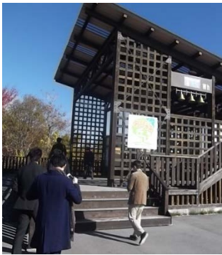
Visitor facility of solar power plant “Mega Solar Iida” constructed in accordance with a power company and Iida City
