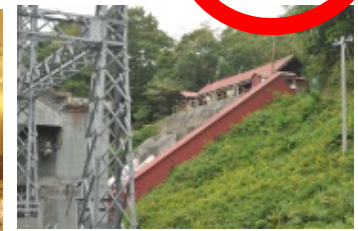
Hydraulic power plant in Niseko town
