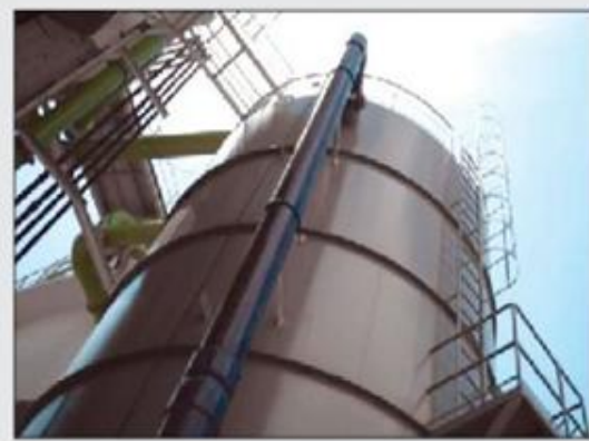
The water is now very pure and is re-mineralised, with lime and carbon dioxide used to adjust the pH level. Chlorine, fluoride and ammonium sulphate are added.
