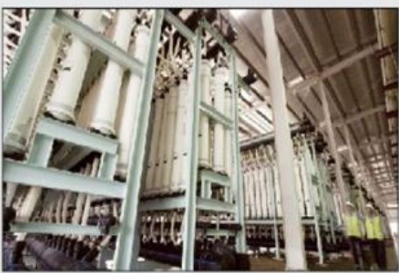
Ultrafiltration membranes are used in desalination pre-treatment to remove micro-organisms and suspended solids in the seawater. The ultrafiltration membranes filter impurities as small as 0.01 micron and block 99.9999% of bacteria.
